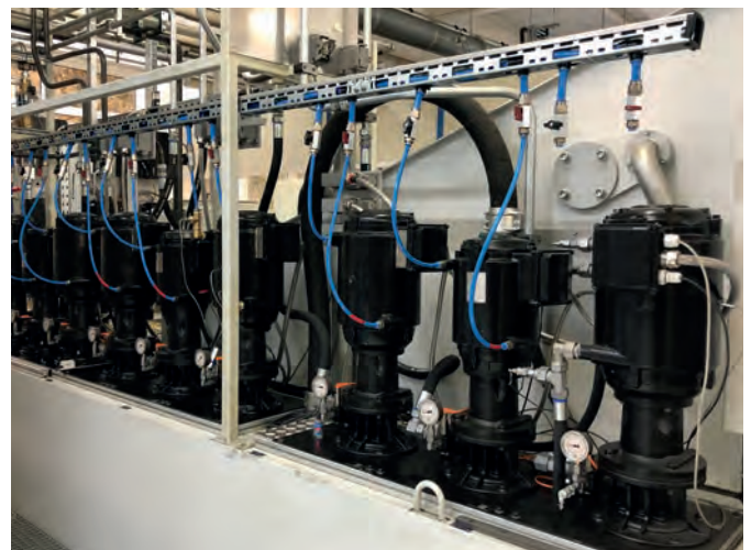
Noise reduction of the system by 8 dB(A) through water-cooled motors, despite the addition of three new pumps at the same time
